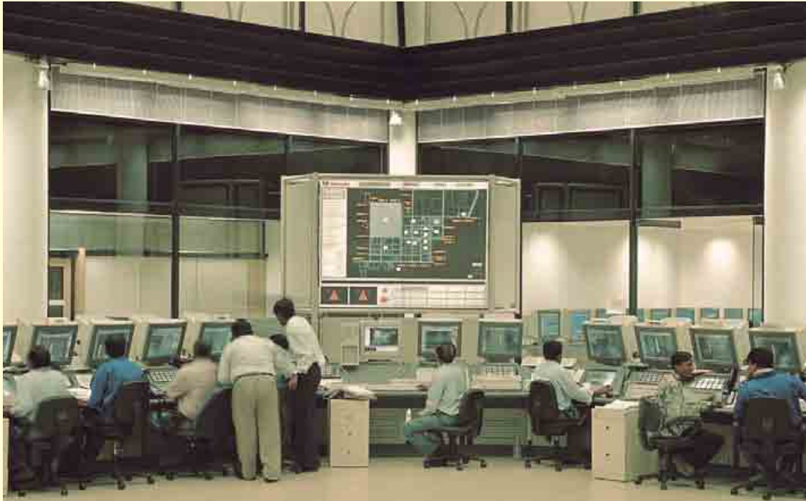
Central Control Room - Distributed control systems for smooth functioning of the Refinery.
